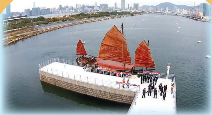
翻新後的跑道公園碼頭 Runway Park Pier after refurbishment works completed
