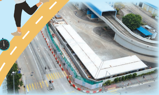
常怡道交匯處的道路擴闊工程 Sheung Yee Road junction widening works
