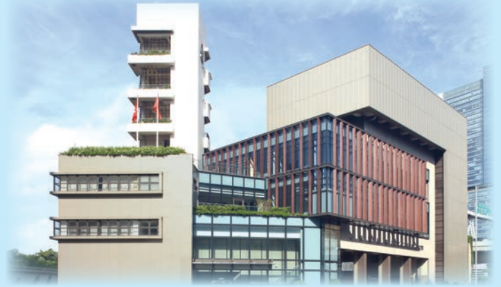
啟德消防局外貌 Outlook of Kai Tak Fire Station
